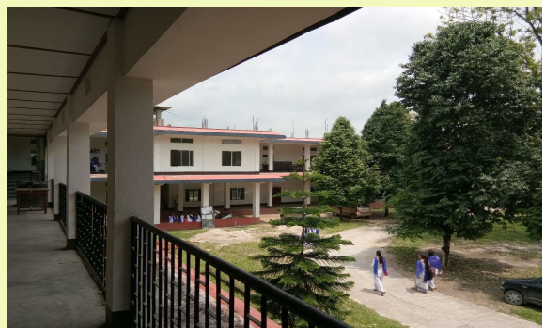
Front view of the Administrative and Departmental Building
